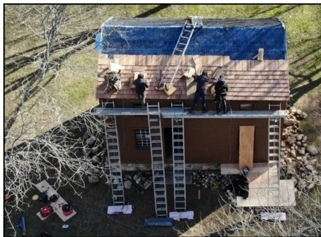
Aerial of new cedar roof installation in November 2023
