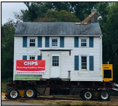
The 1713 East Jersey Cottage being moved and placed in its new location in Millstone Park, October 2019.
